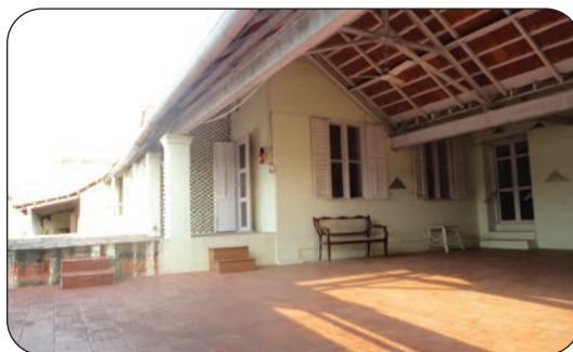
The 'Roof' at the Headquarters building
