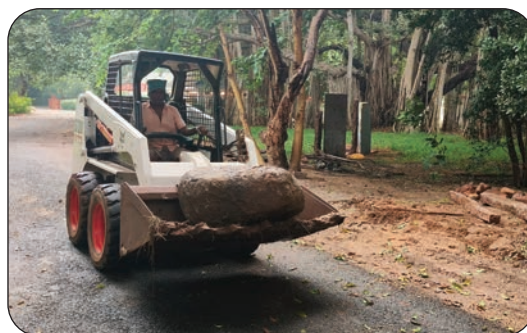
The handy 'Bobcat' moving boulders on the estate
